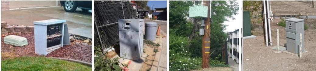
**Figure 2 - Example cable broadband powering sites. The variability in available space, loading, and local regulations makes a one-size-fits-all solution for ESS solutions nearly impossible.**
