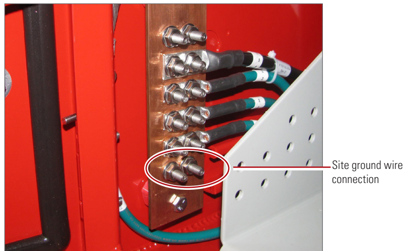
Figure 10: Enclosure MGB and chassis ground
