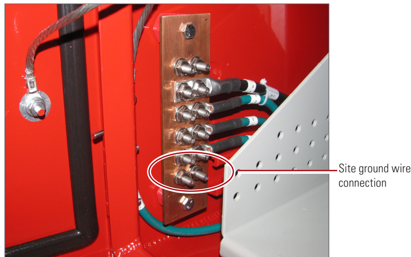
Figure 10: Enclosure MGB and chassis ground
