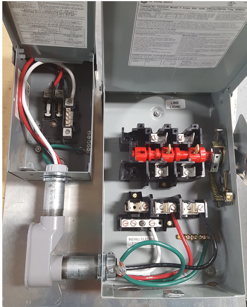
Fig. 5, Complete Wire Installation
