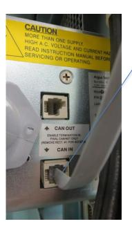
CAN cable from L-ADIO on a Single Rectifier Shelf system.
