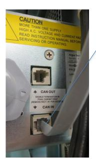
CAN cable from L-ADIO on a Single Rectifier Shelf system.
