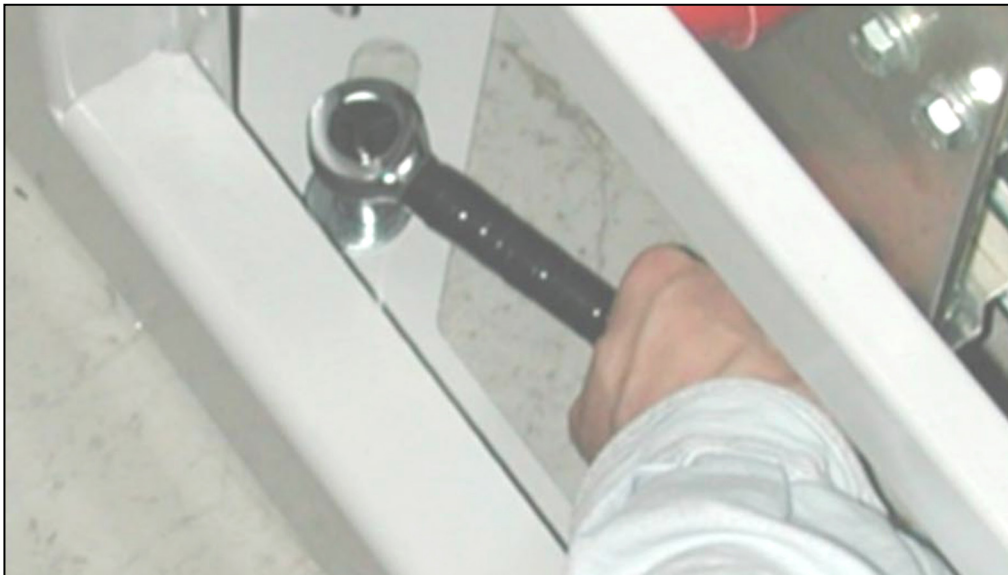
Figure 14 — Securing power system bay to concrete floor
