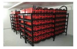
Figure 3: Racks of TPPL-based EnerSys® PowerSafe® batteries providing back-up power in a subsea fiber optic cabling application
