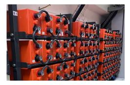
Figure 2: EnerSys® PowerSafe® battery strings with TPPL technology installed for backing-up mobile network infrastructure
