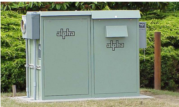
Figure 3: Typical Curbside Generator Installation Using Natural Gas
